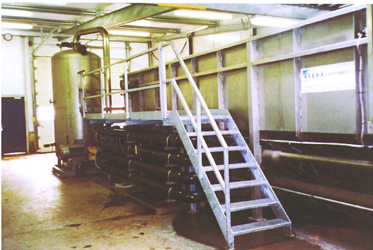
Fig. 6 Flotation system, type WWL 180, for flotation of e.g. activated sludge
